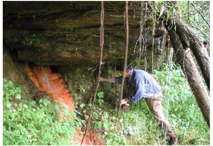
Water seeping from the bottom of a coal sludge impoundment in Mingo County. A private party had the water tested—it has high levels of mercury. The water flows into a creek which empties into the Tug Fork.
